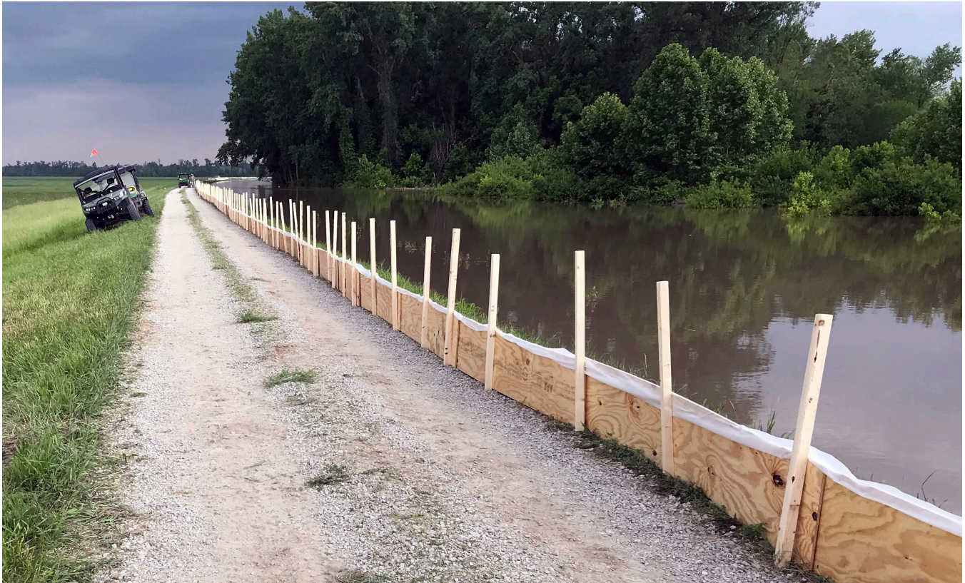
Figure 20: Lumber and poly sheets used in the construction of flashboard
