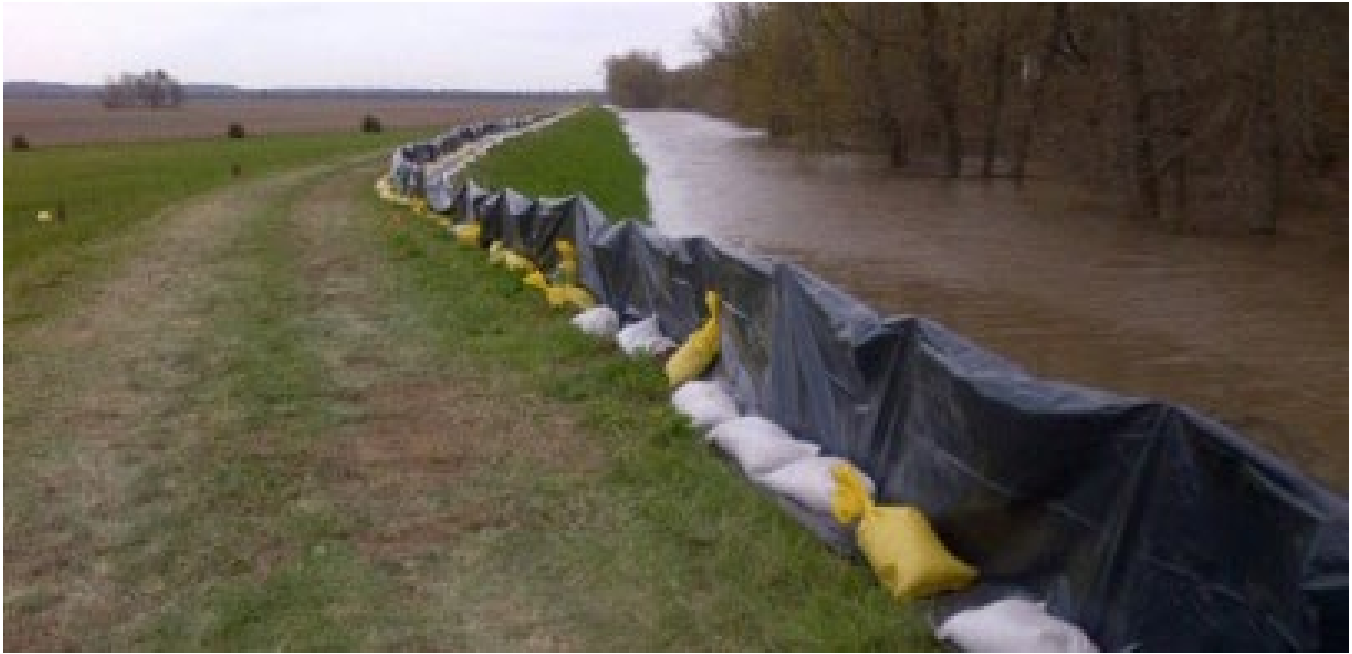
Figure 24: Flashboard installed along levee crest
