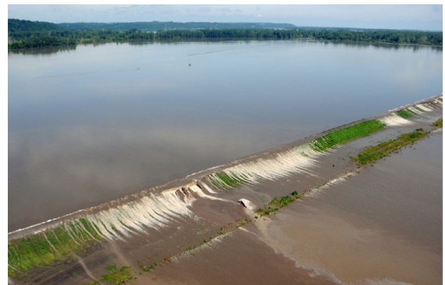
Figure 22: Overhead photo of levee overtopping
