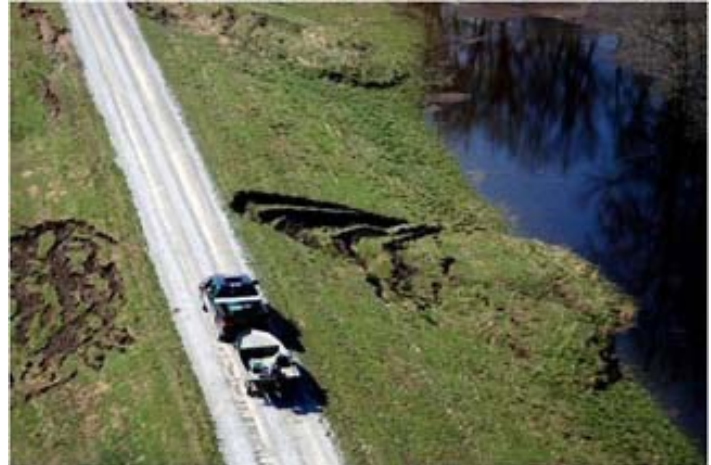
Figure 31: Image of levee embankment slide
