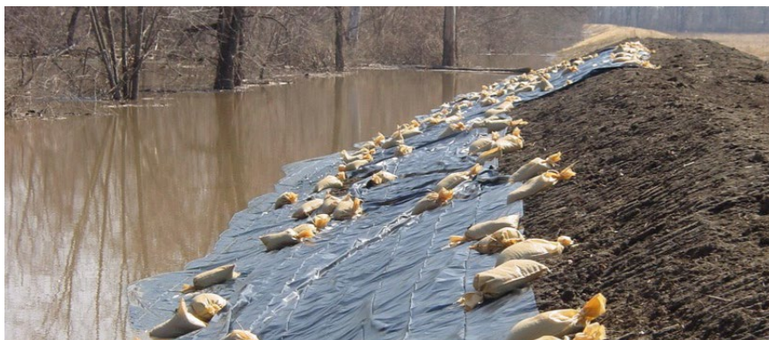
Figure 17: Poly sheets used for levee armoring
