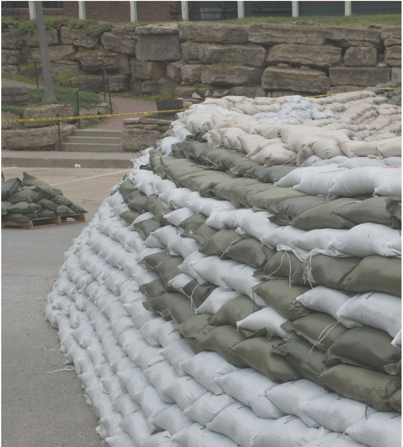
Figure 12: Sandbags placed into a temporary dike
