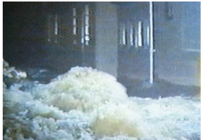
d: Very Large, Very High Activity, Concentrated Leak under floodwall
