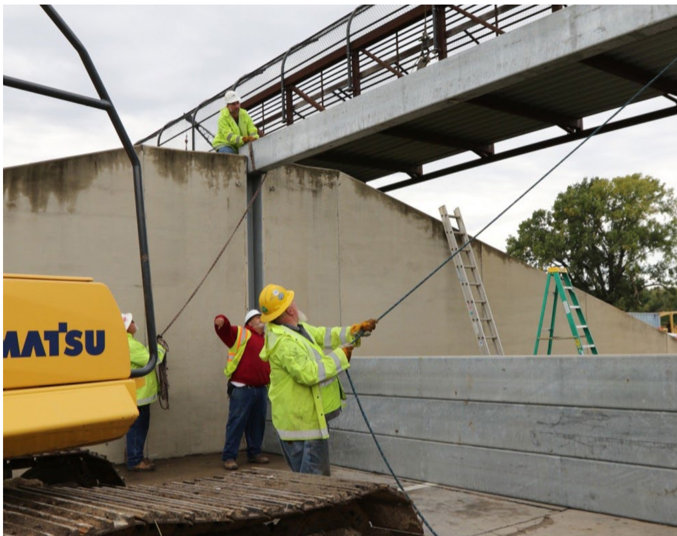
Figure 33: Installation of wooden stoplogs being slotted into place at gap closure
