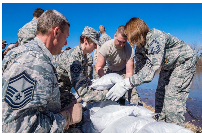
Figure 23: Sandbag capping (Credit: 139th Airlift Wing)
