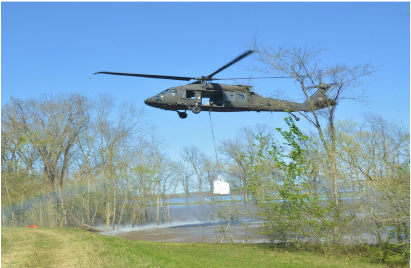
Figure 15: Super sandbag being delivered by helicopter
