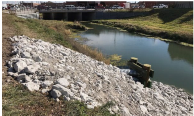
Figure 29: Levee damage repaired with rip rap
