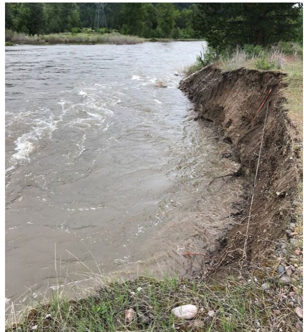
Figure 28: Image of levee scour
